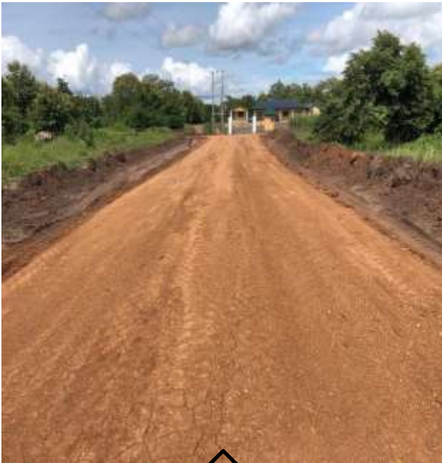
Opened and Graveled 0.68km Road to Ginger Factory at Chiranda
