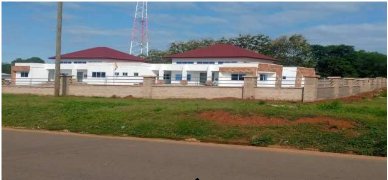
Completed and Walled Court Building in Kintampo
