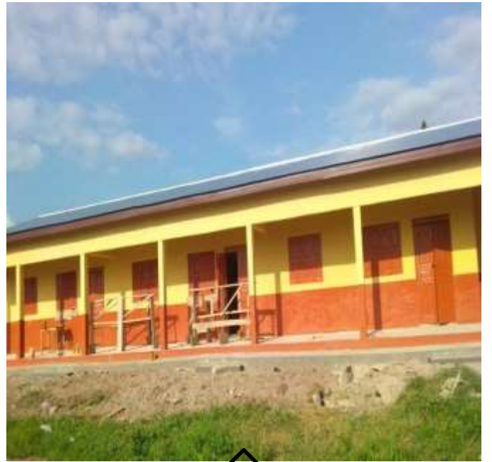
Completed and furnished 3-Unit Classroom Block with Auxiliary Facilities
