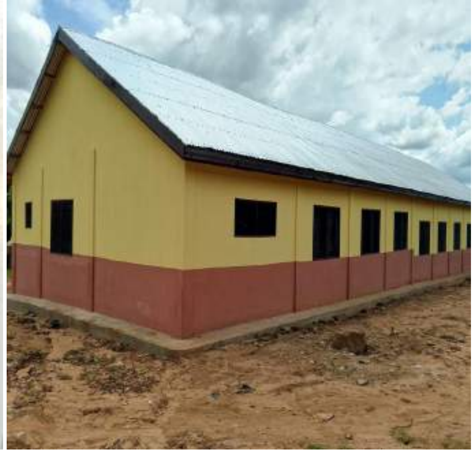
1 No. 3unit classroom block with office, store and Girls changing room-SDA
